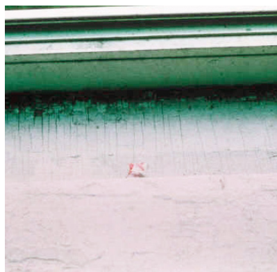
FIGURE 5.4b Alligatoring paint
