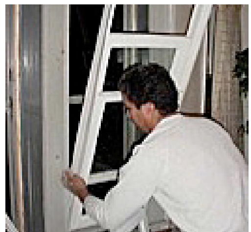
Figure 11.14 Reinstall sash into jamb.
