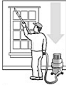
FIGURE 14.10 The HEPA Vacuum-Wet Wash-HEPA Vacuum Cycle Helps Meet Clearance Standards.
