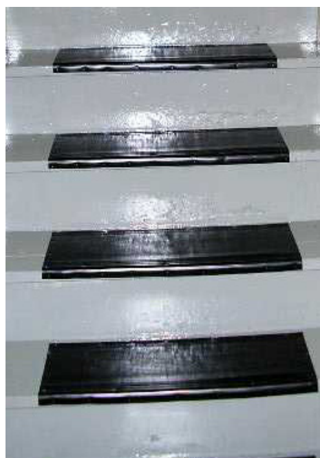
FIGURE 5.6b Friction hazard on stairs post-treatment.
