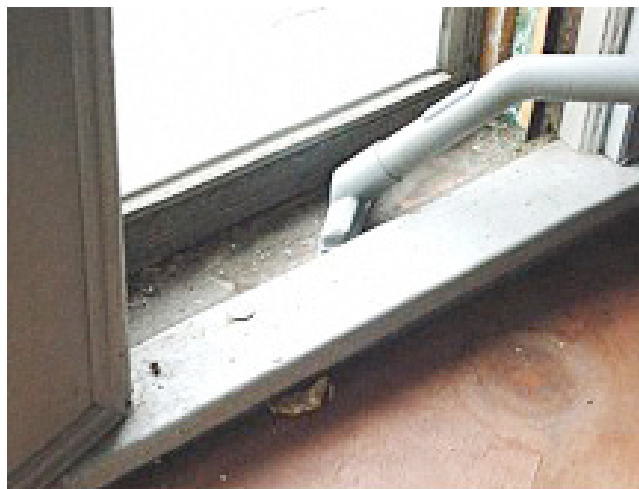
FIGURE 11.5 Prepare the worksite and pre-clean the window.
