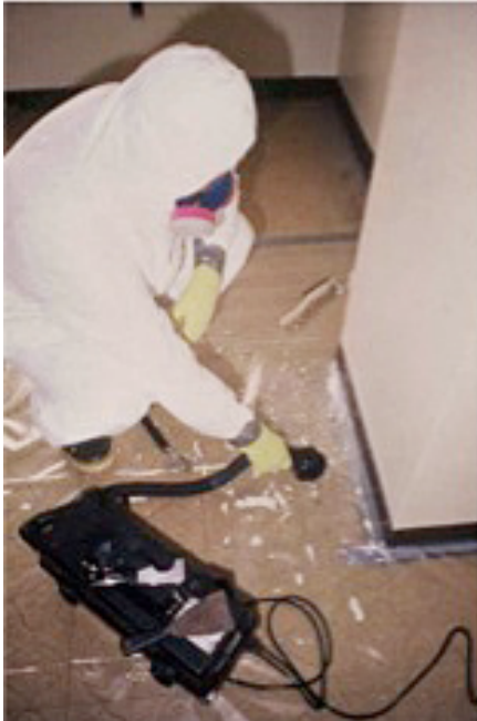
FIGURE 14.8 Vacuuming the floor containment.
