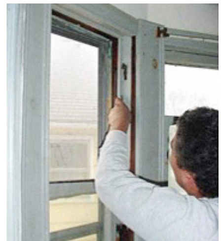
FIGURE 11.6 Remove parting Ahead.
