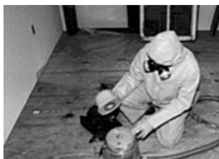
f) Remove & Replace HEPA Filter Assembly.
