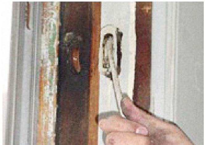
FIGURE 11.8 Remove sash controls/weights.
