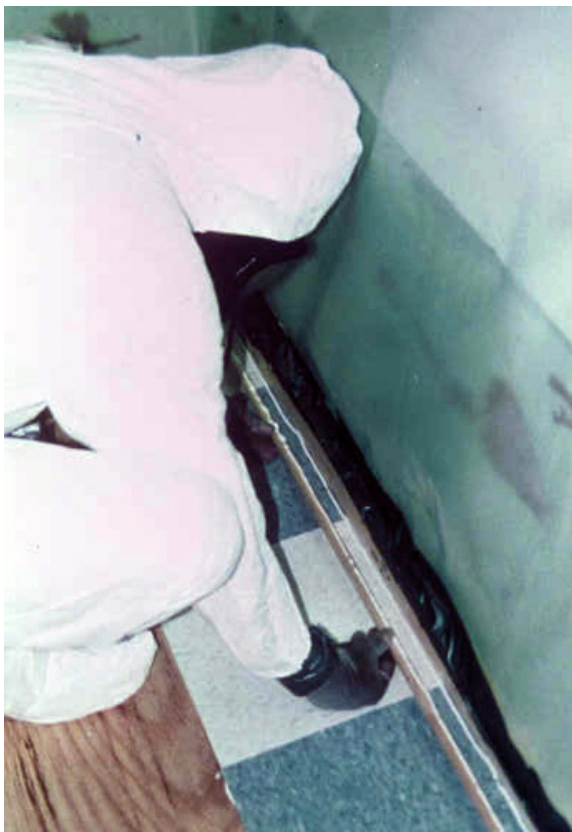
FIGURE 13.1 Encapsulating a floor with vinyl tiles
