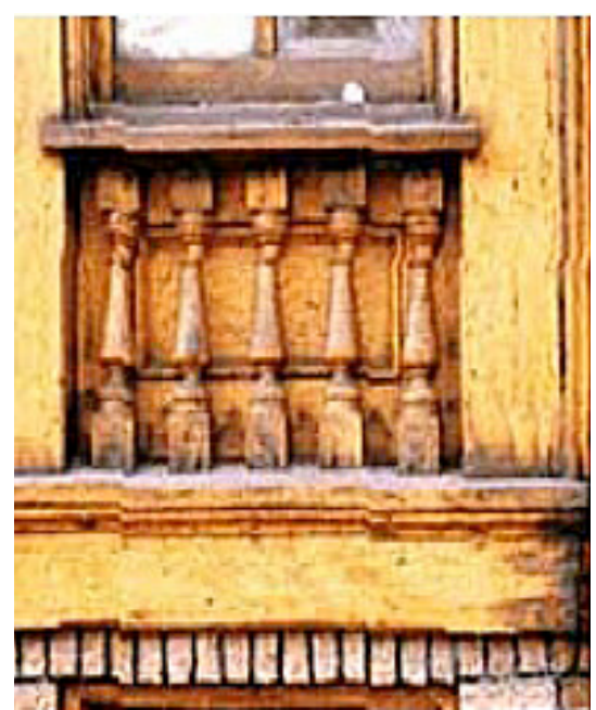
FIGURE 18.4 Wood features on historic properties. Sometimes they can be stabilized instead of stripped of traditional painted finish as in this photo. Photo courtesy of National Park Service.
