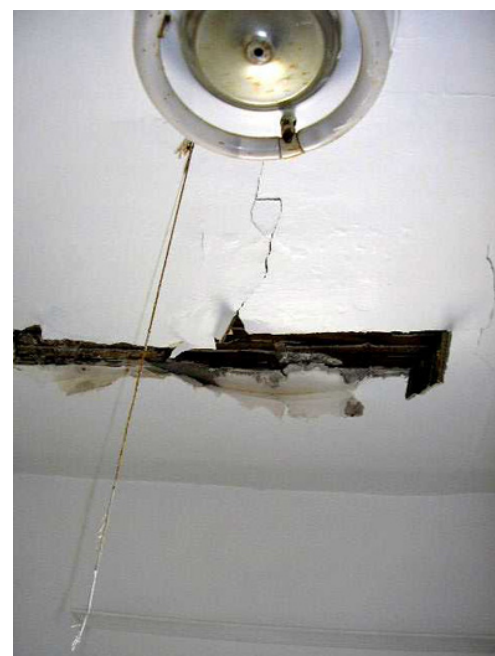
FIGURE 8.4 Example of structural deficiency needing repair prior to work.
