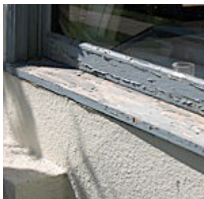
FIGURE 5.4a Peeling paint
