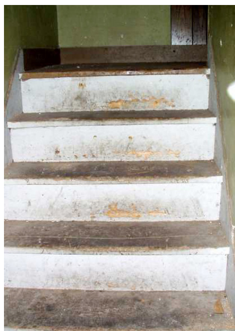
FIGURE 5.6a Friction hazard on stairs pre-treatment.
