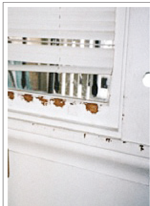
FIGURE 5.8 Chewable surface: teeth marks on window sill.
