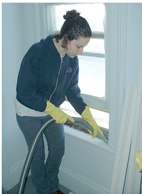
FIGURE 8.17 Pre-cleaning window with HEPA vacuum.
