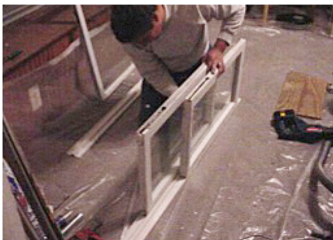
Figure 11.13 Fit sashes into jamb liners.
