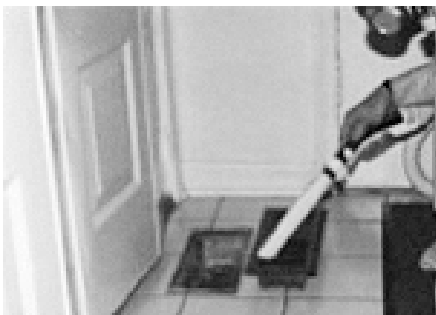
a. Vacuum and remove register covers;
