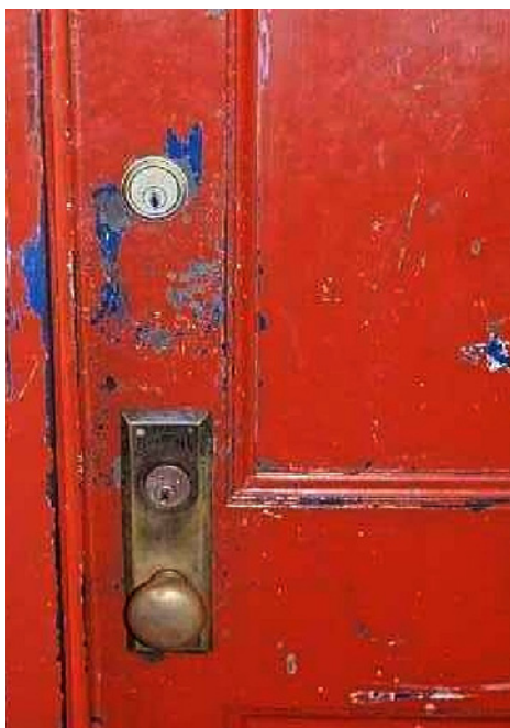
FIGURE 1.3 Paint deterioration.
