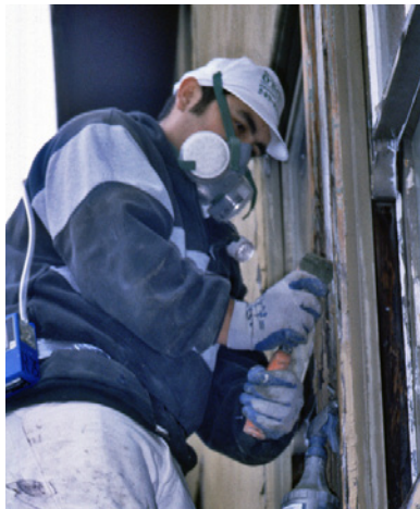
FIGURE 12.16 Wet scraping (left)
