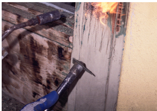
FIGURE 4.2 Torching and burning old paint is a prohibited work practice that can generate lead fumes.
