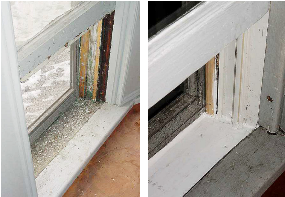
FIGURE 11.3 Window before and after friction treatment.
