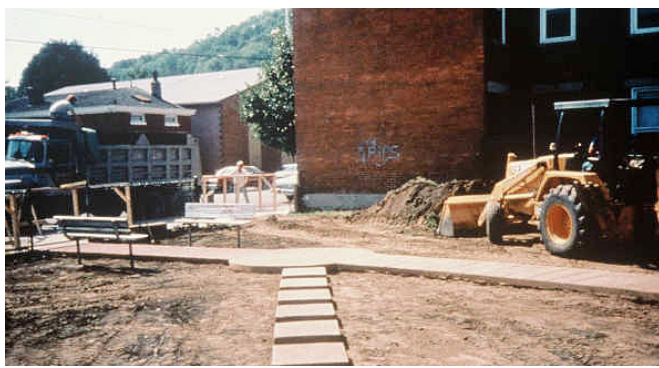
FIGURE 12.22 Replacing resident pathway after soil removal.
