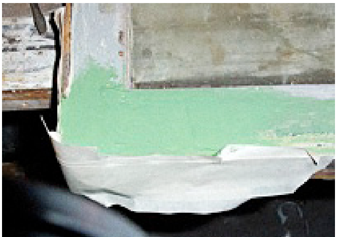
FIGURE 11.10 Rebuild damaged sash with filler or putty.
