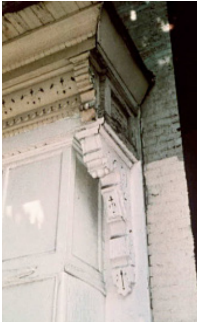
FIGURE 13.3 Encapsulated historic components.
