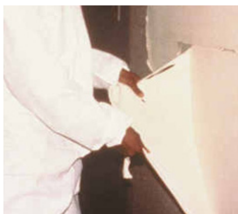
FIGURE 13.4 Encapsulant failure.
