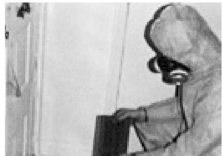
c. Wet wash register covers and replace
